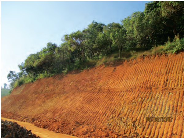
This photo was taken on February 17 th 2017 in Ba--- village, Ta Naw Th’Ree Township, Mergui-Tavoy District. It shows construction workers build a road on the land of Saw Az---, a local villager shown in the photo on the right. Because the construction workers dumped soil and rocks on his land, they damaged 300 cashew trees and 500 rubber trees on Saw Az---’s land, threatening his livelihood. [Photo: KHRG] 213
