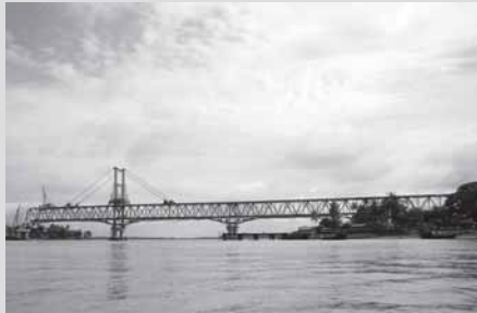
The bridge while under construction
