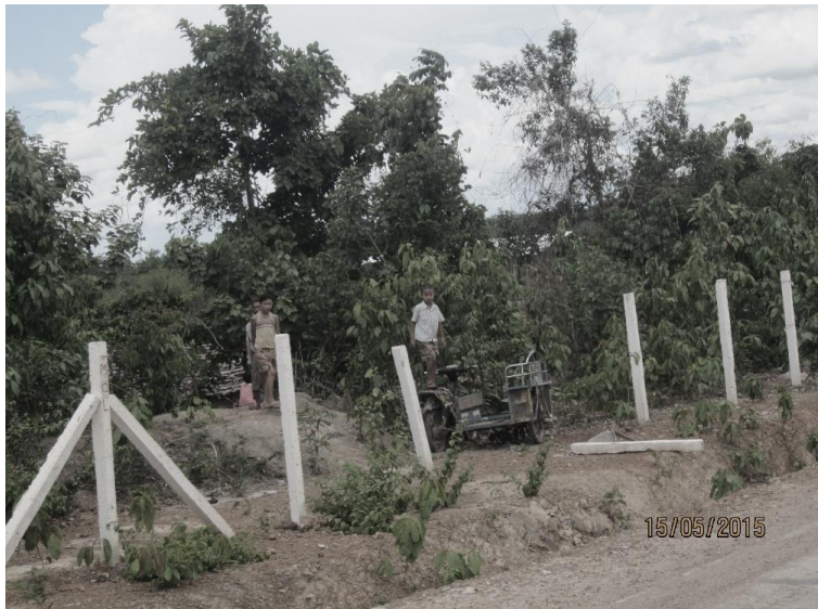
Figure 26: MCL fence which blocked an existing road. Local farmers had to move the fence in order to use the road
