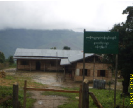
Primary school (1-6 grades) were built by local Authority and villagers
