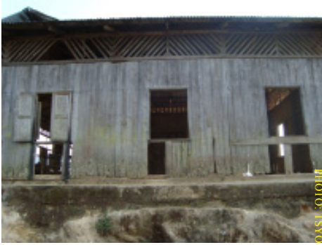
School in urgent need to repair
